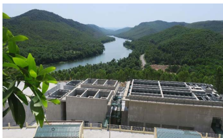
Drinking water treatment plant in Quang Binh province, Vietnam Capacity: 10,000 m 3 /d Budget: 10€ million
