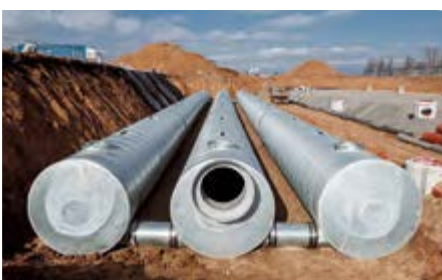
Stormwater solution for NEXEN Tire plant in Žatec (Czech Republic) 1,200 m 3 of corrugated steel pipes
